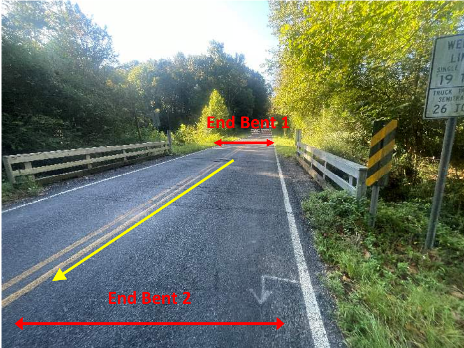
Photograph No. 1: View looking north at End Bent 1 from End Bent 2
